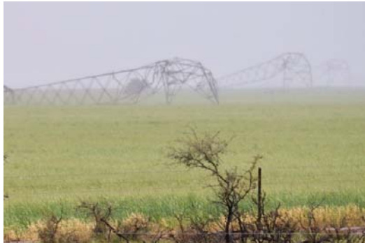
Above: Damaged transmission lines in South Australia in 2016
