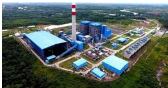
Mine Mouth Power Plant (PLTU Sumsel 8 - PTBA)
